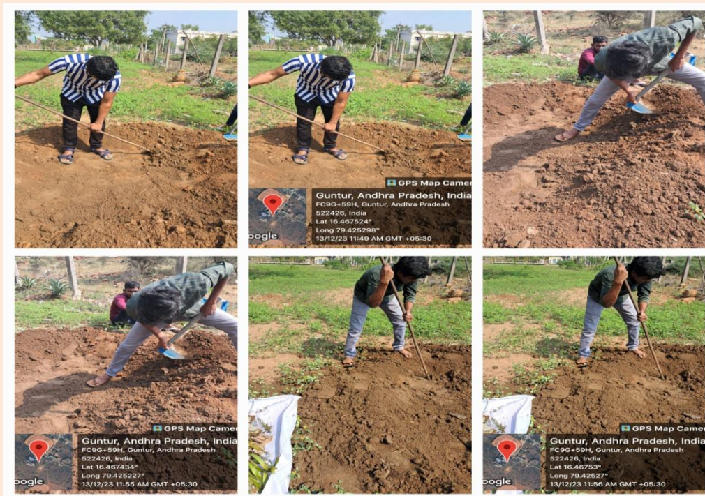
Preparation of a pit for dumping of the solid waste, collected from the college campus
